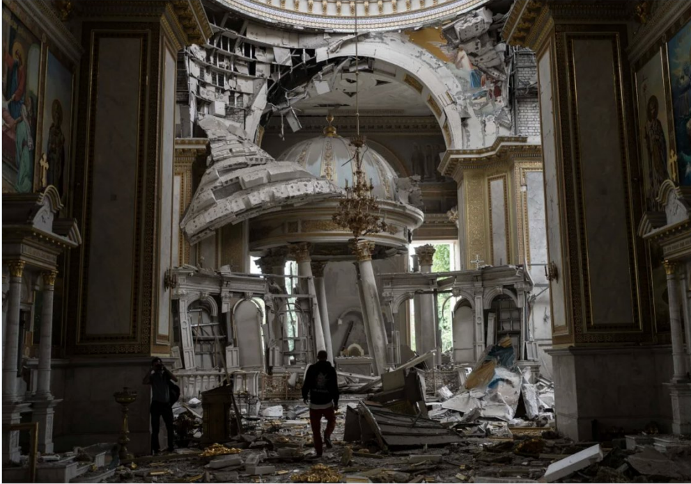
Church personnel inspect damages inside the Odesa Transfiguration Cathedral. Jae C. Hong/AP
